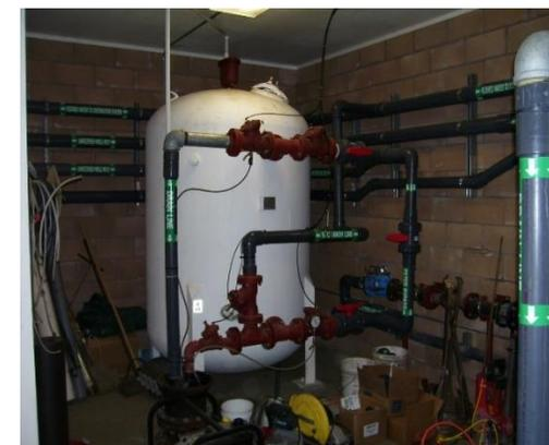
Greensand filter to remove iron & manganese
